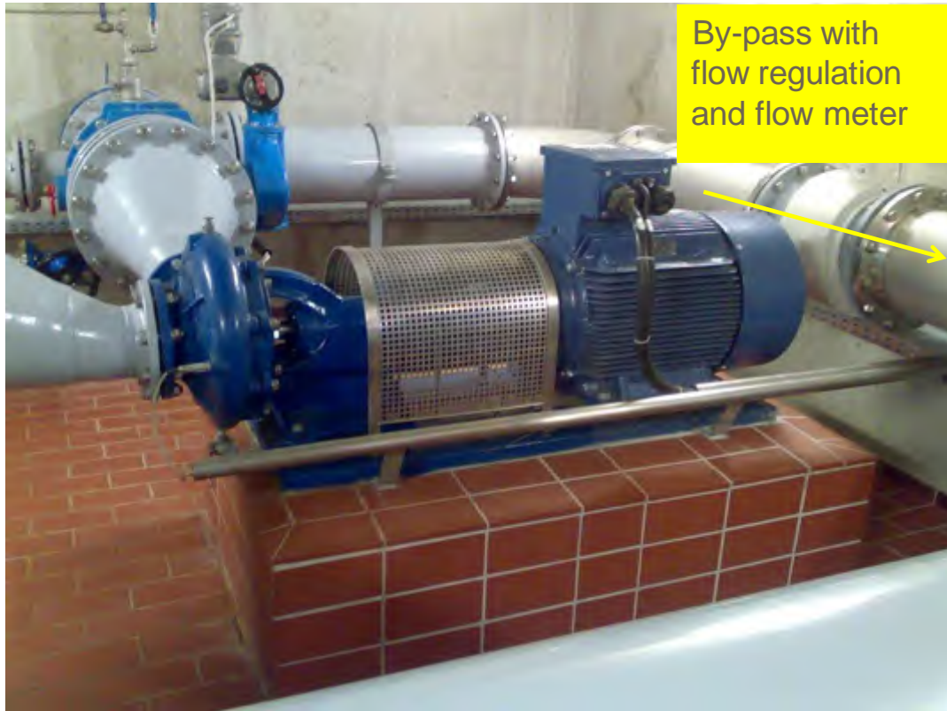
Figure 16 WW Stellingen: Pump as Turbine
