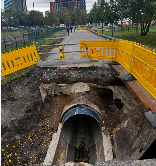
Facilitated insertion of the Alphaliner1800H DN 1800 by using a conveyor belt with folding device.
