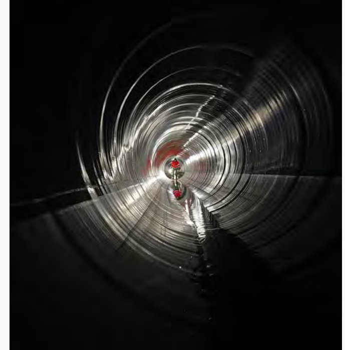
As far as the eye can see: a total of 1,000 metres of old pipe rehabilitated.
