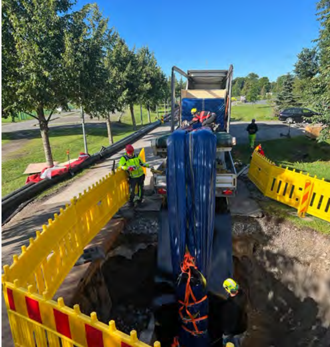
Facilitated insertion of the Alphaliner1800H DN 1800 by using a conveyor belt with folding device.
